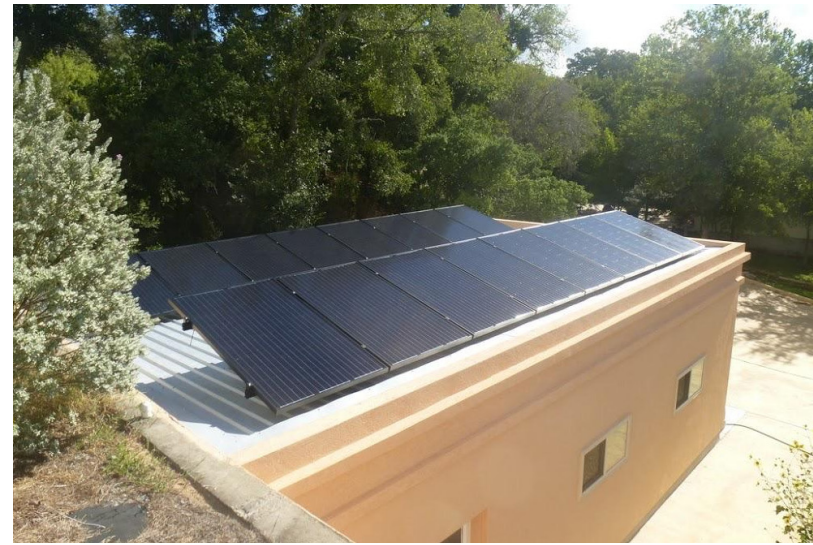
Tilted, Flat-Roof Mounted SED (Bastrop, Texas)
